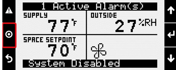
2. Press the Enter button on Ctrl Variables to access the Ctrl Variables Menu.
