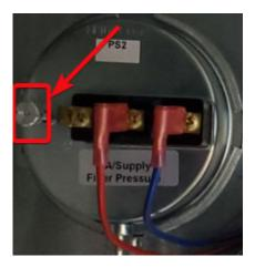
2. Rotate the knob until the dirty filter alarm clears. The direction of rotation may vary depending on switch model. Once the alarm has cleared, verify that the switch is now open across its terminals. Once the alarm clears and the switch opens, rotate the knob one more full turn to increase the trip point.
