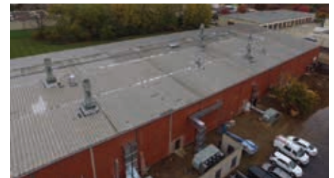
Promerus roofline after renovations.
