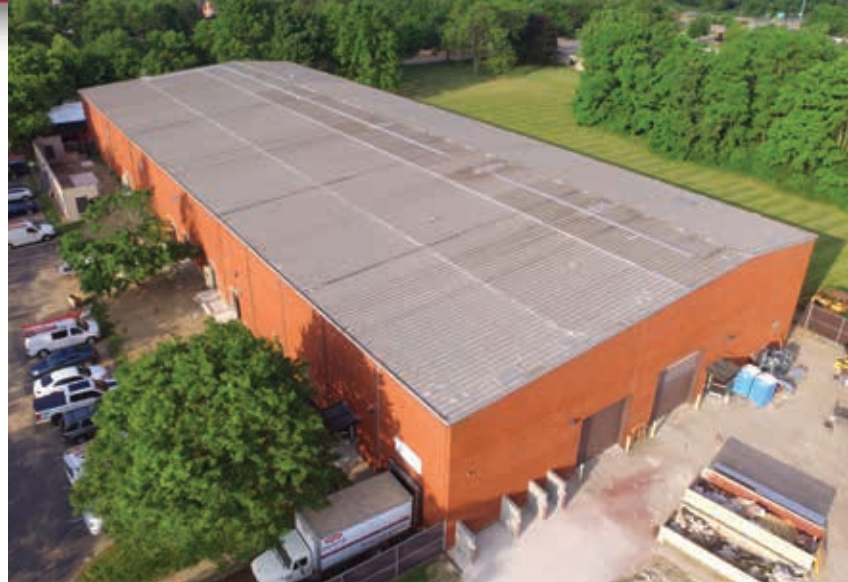
Promerus 38,000 square foot building prior to renovation.
