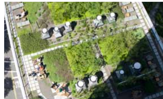
Residents relax on the Solaire rooftop with greenery and Greenheck fans.
