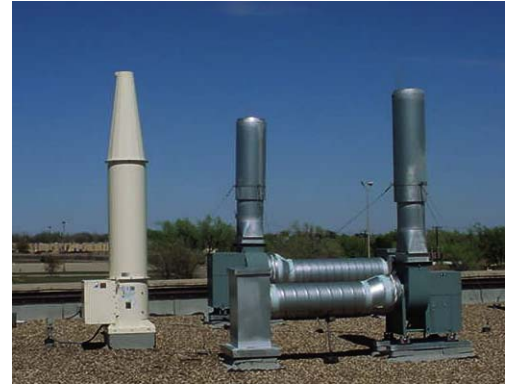
The TCB-LE shown on the Texas Tech University project. This unit is suitable for flow applications from 500 to 24,000 cfm per fan,
