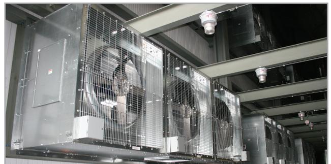
Greenheck's custom-designed special direct drive "Utility Duty" propeller fans in a 90" x 90" wall housing
